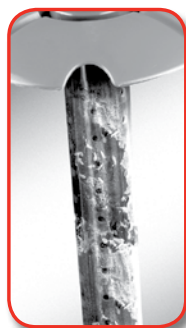
Termites are present inside the stake
