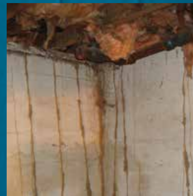
Mud tubes along the concrete wall of this damp basement allow termites to travel into the home above.
